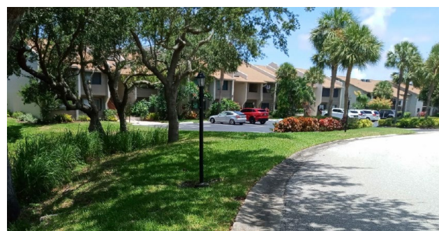
South Side Looking West
